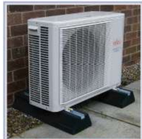
Mounting a condensing unit
