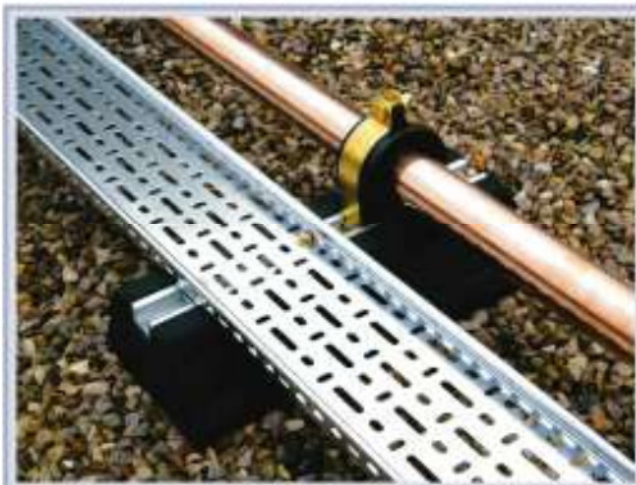
Supporting cable tray and pipework
